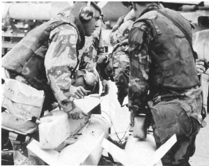
Marine ground crewmen prepare to load a HARM anti-radiation missile on an F/A-18 Hornet strike fighter. Marine ground crews wore their flak jackets and carried their gas masks on the flight line.
